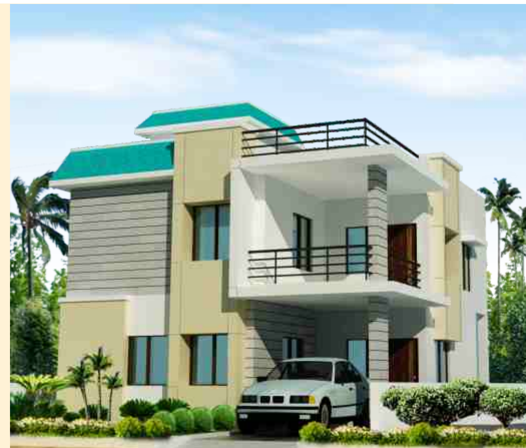
South Facing Villa
